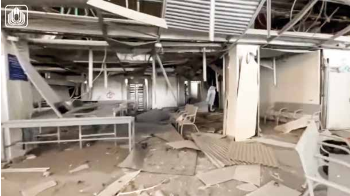
Damage to Erez crossing between Gaza and Israel, October 2023. Photo credit: Israel's Ministry of Defense Press Office.
