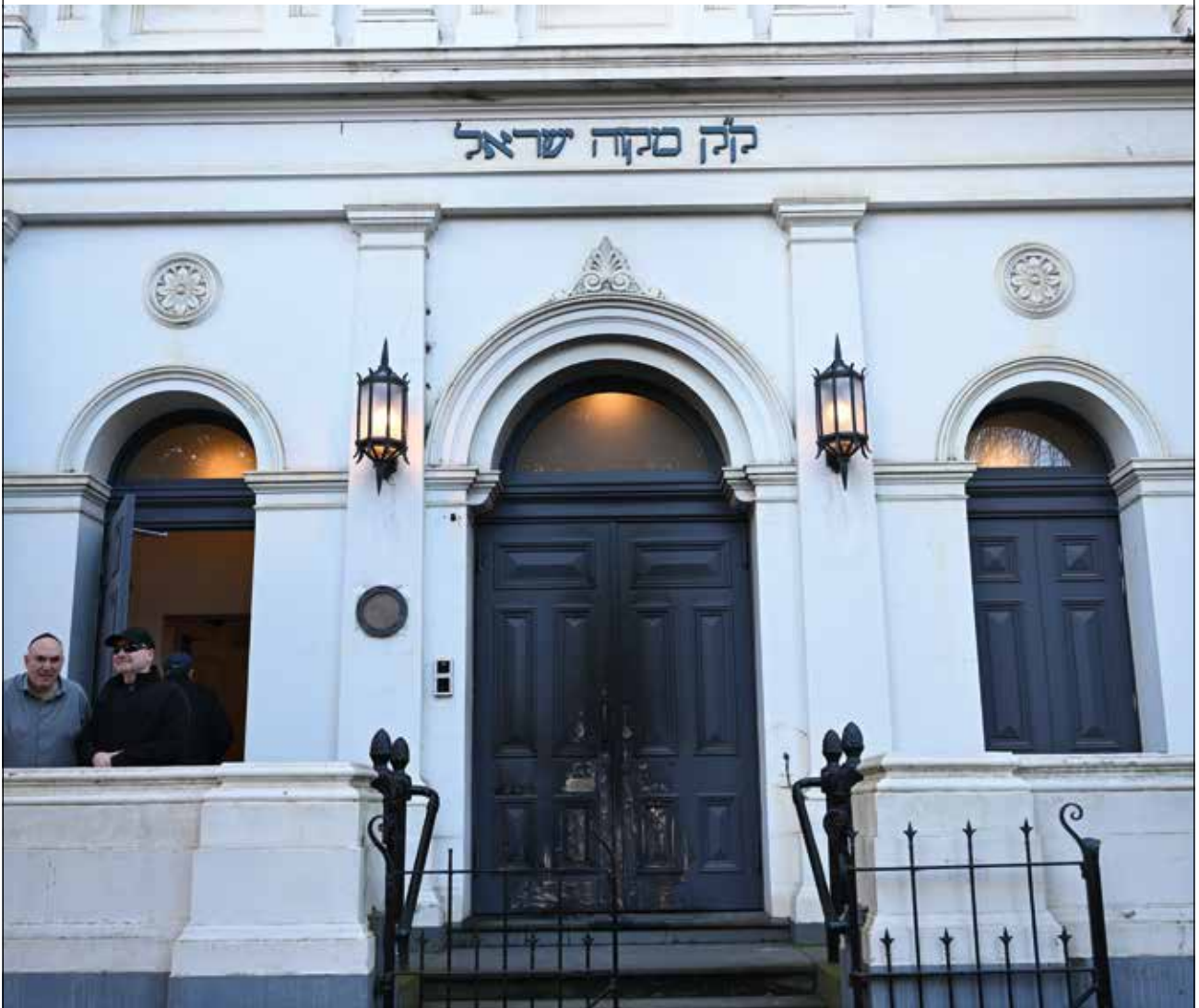
A view of the damaged exterior of the East Melbourne Hebrew Congregation in Melbourne, Australia, July 5, 2025. Photo credit: via Reuters
